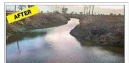
The same nullah, full of water, in May 2021
